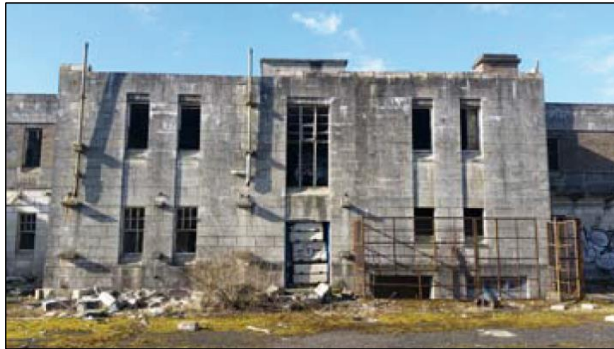
Figure 5.2: North elevation of Officers Mess building
